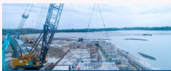
Pekerjaan Capping Beam/Capping Beam Work
