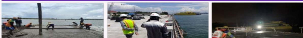
Pengecoran Pelat Lantai, Pembesian Kansteen, Curing Plat Lantai Floor Plate Casting, Kansteen Wireless, Floor Plate Curing
