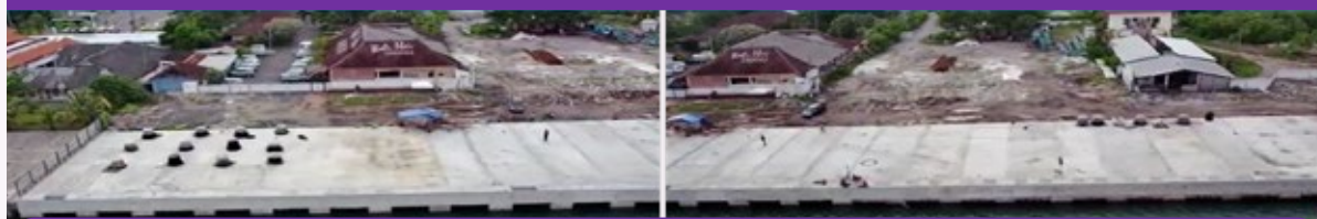
Aerial View Pekerjaan/Aerial View Work
