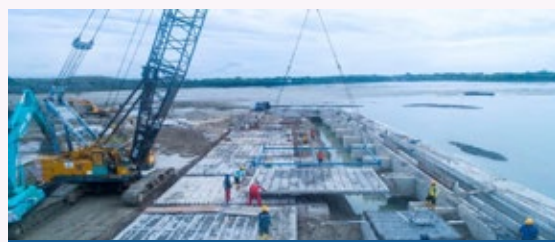
Pekerjaan Instal Halfslab/Halfslab Install Work
